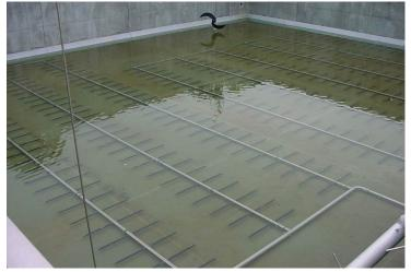
ENVICON EMR membrane tube diffusers are quality products manufactured in Germany. Sophisticated membrane mixtures, a modern production process, together with optimised fine-bubble perforation guarantee a high-quality product throughout their service life and durable, cost-effective operation of aeration systems.
