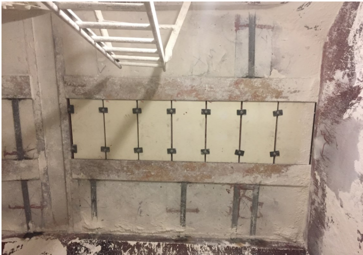
The frame, complete with seven new tiles, installed into the sloped floor of the 'kettle hot pit'.
