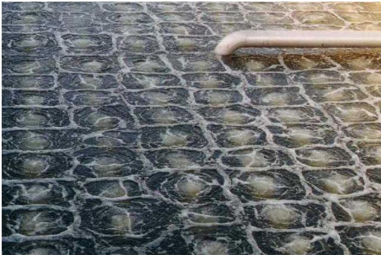
Measurements were taken under standard conditions according ATV M209 (clean water, water depth = 4,0 m, density of aerators 1,1 pc. EMS / m<sup>2</sup>)
