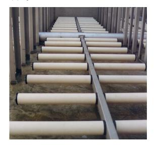
Mantec's ceramic tube diffusers are available in various lengths and diameters and are usually supplied without fittings. However, fittings can be offered upon request.
